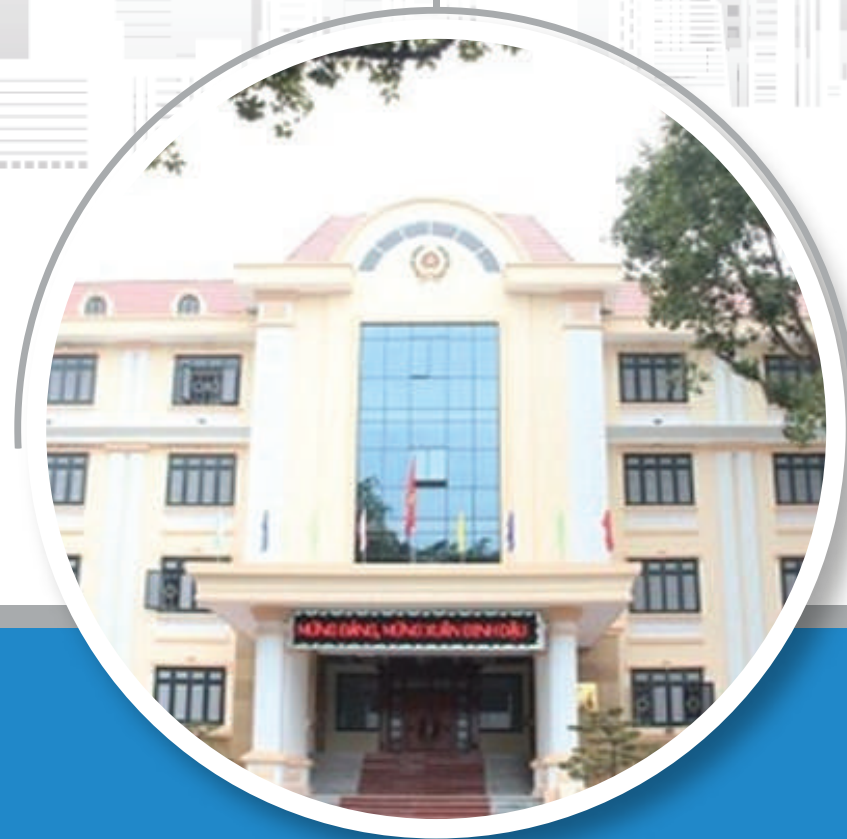
Implementation of network, telephony, television, and fire alarm systems at Hiep Hoa District People's Committee
