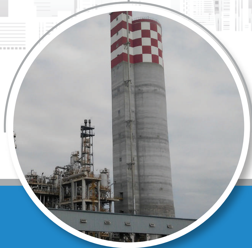
Supply of equipment and installation of camera systems for workshops at Ha Bac Fertilizer Plant
