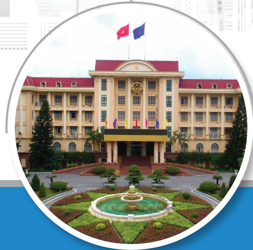
Implementation of network, telephony, television, CCTV, and public address systems for Bac Giang City People's Committee office complex
