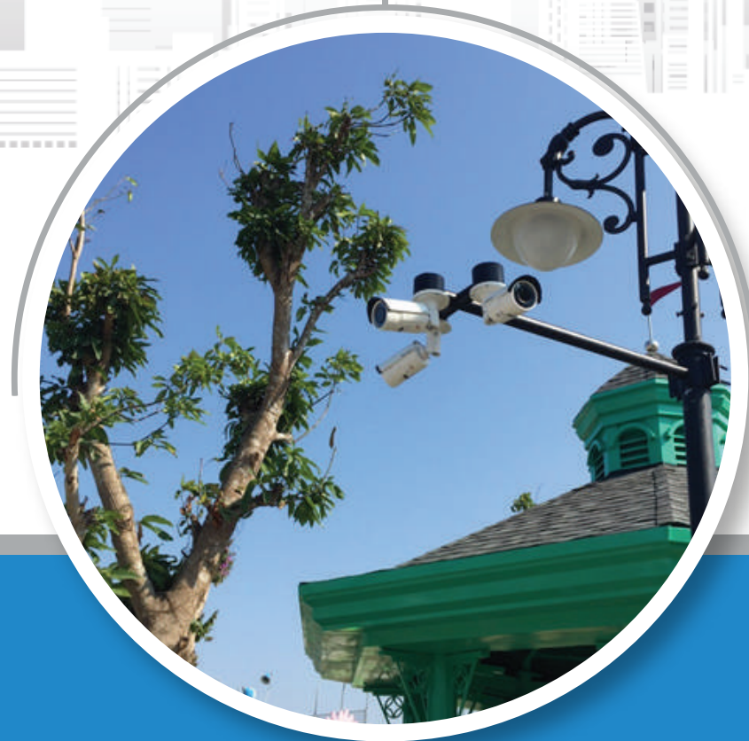
Installation of surveillance camera system at Vinpearl Nam Hoi An
