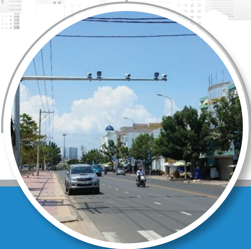
Installation of 29 security surveillance camera points across Bac Giang City
