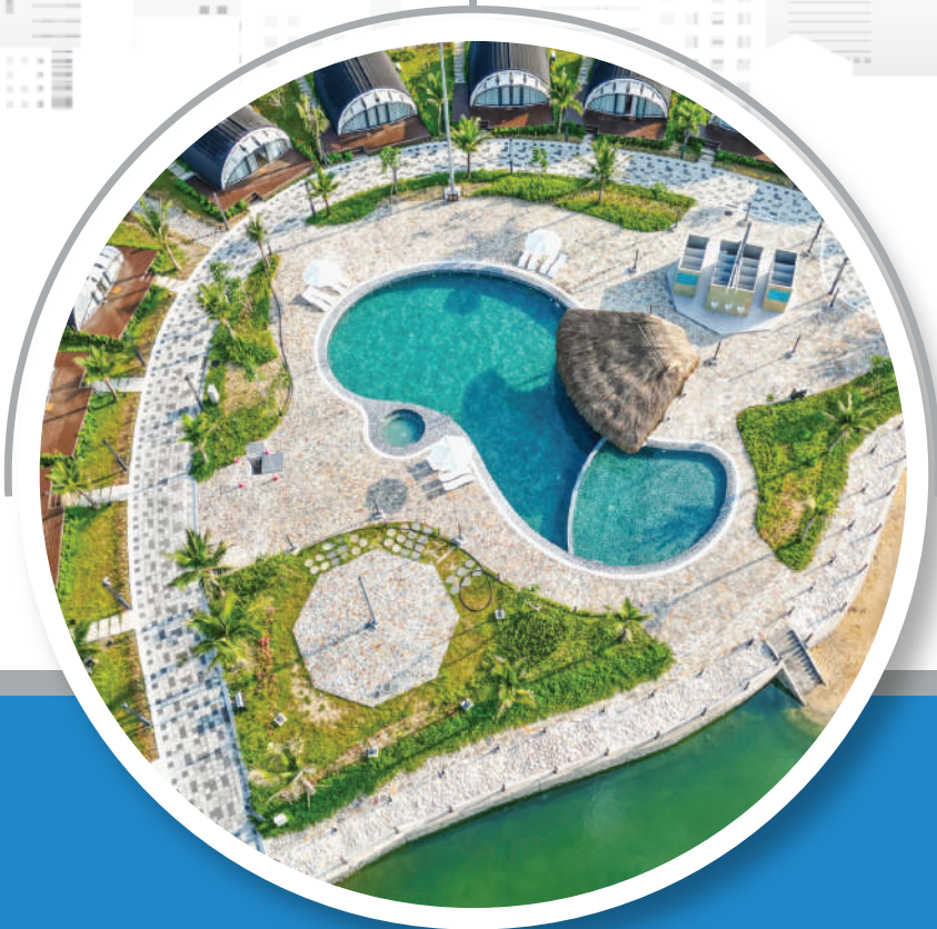
Design, supply, and installation of network infrastructure, CCTV, and audio systems at Dau Rong Entertainment & Resort Complex
