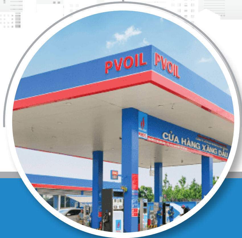
Supply and installation of CCTV systems for fuel station chains across Bac Giang Province
