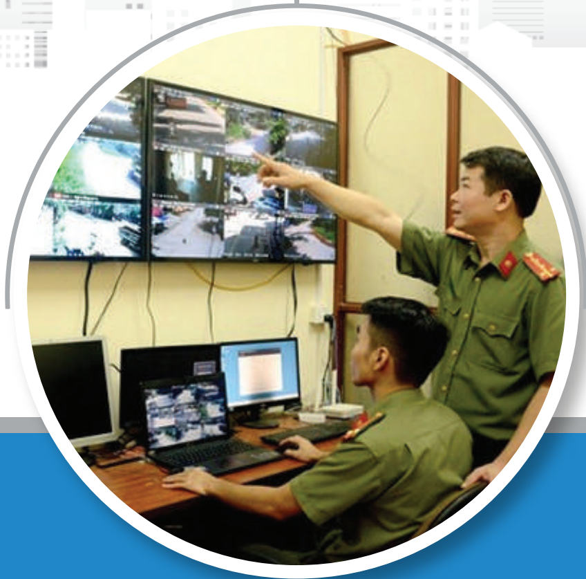
Installation of security surveillance camera systems in Viet Yen District, Bac Giang Province
