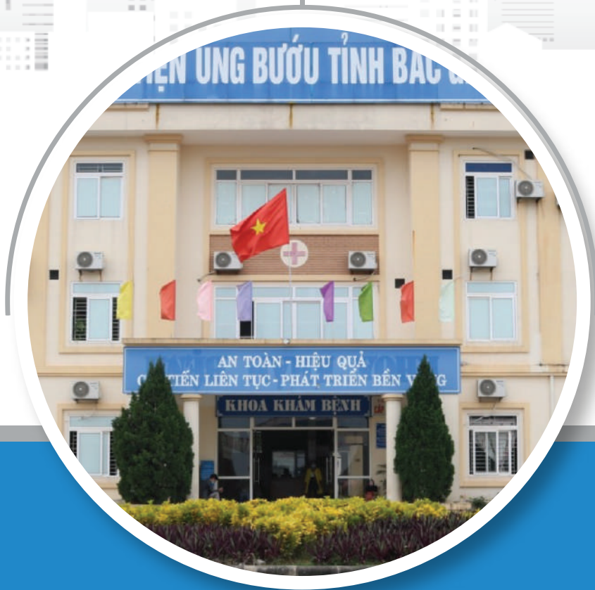
Implementation of network, telephony, television, nurse call system, and fire alarm system at Bac Giang Oncology Hospital
